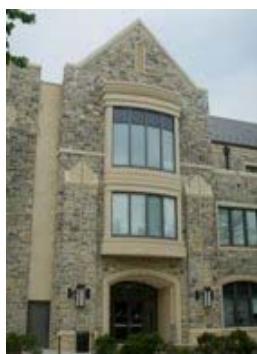
Student Services Building
